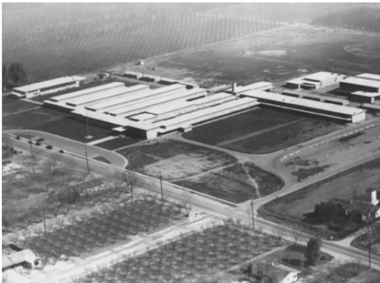
Thomas Downey High School prior to its opening in 1951. Note the surrounding orchards as well as the absence of the auditorium, student center, girls' gym, government building and western classroom wings.
